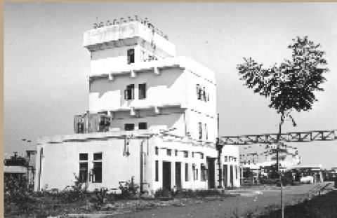
CHEMICAL PLANT - TUNGSTEN ORE TO APT
