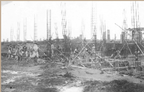
FACTORY BUILDING CONSTRUCTION
