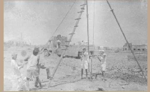
PILING-BEGINNING OF CIVIL CONSTRUCTION
