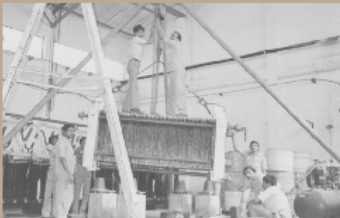
INSTALLATION OF MACHINERY
